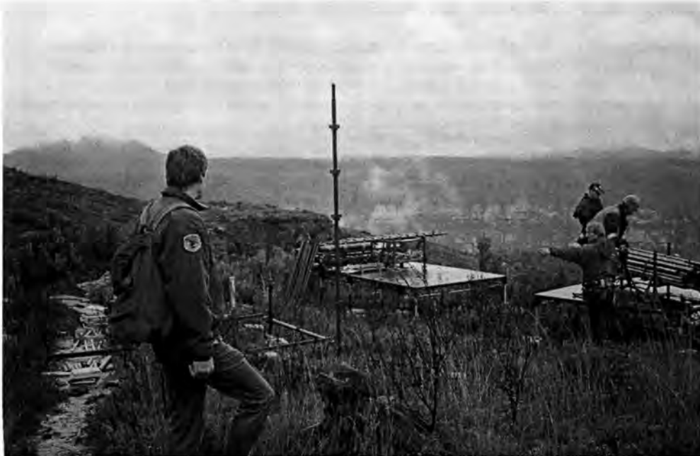
Partially completed camera platform at Butterbox Point supervised by NPWS (Grose Wilderness) (Courtesy: Sue Morrison)
